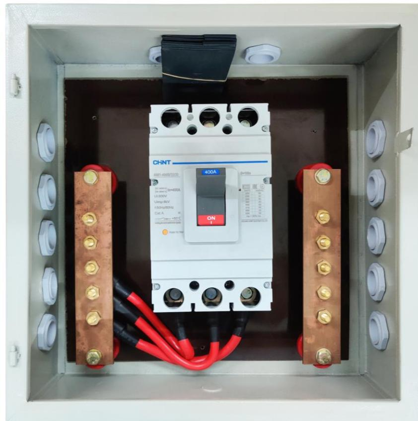
**BusBar for 3 inverters in parallel**
