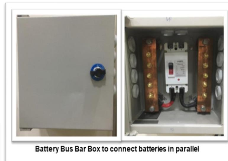
**Battery Bus Bar Box to connect batteries in parallel**
