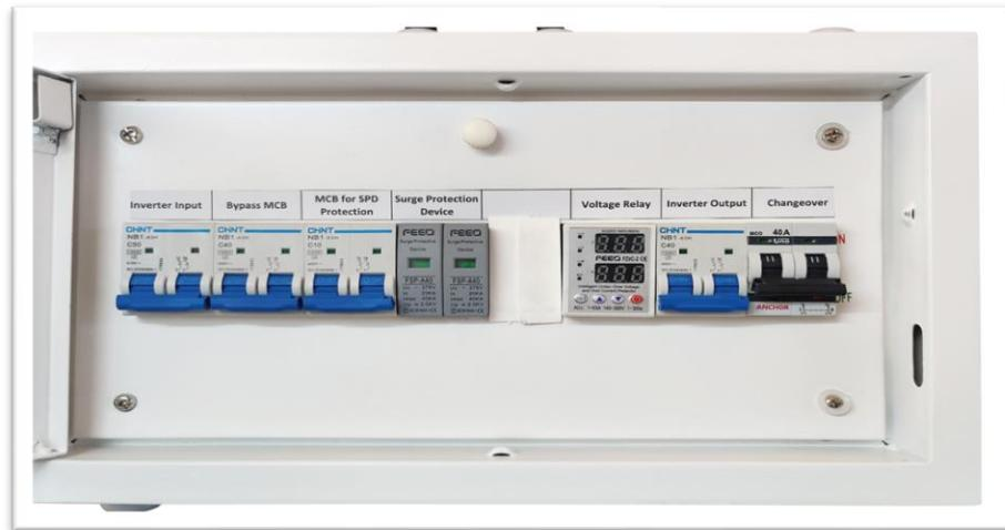
**AC Prewired Box: Comes with 3 x DP AC MCB, 1 x 10A DP AC MCB, 1 x Voltage Regulator, 1 x 2P AC SPD, 1 x 40A Changeover and earthing terminal.**
